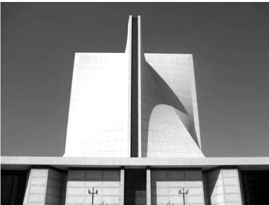
Fig. 15: Pier Luigi Nervi, with Pietro Belluschi and McSweeney, Ryan and Lee Architects – St. Mary Cathedral, San Francisco, 1963–1971
