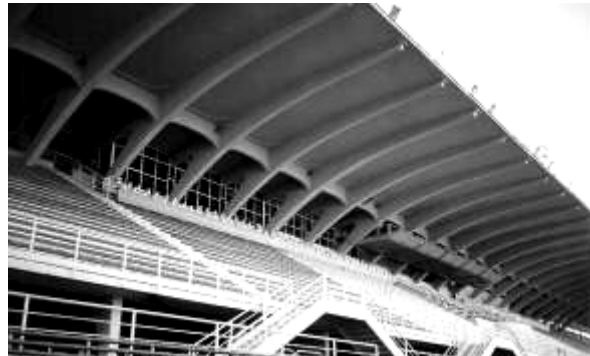
Fig. 2: Pier Luigi Nervi – Municipal Stadium, Florence 1930-32
