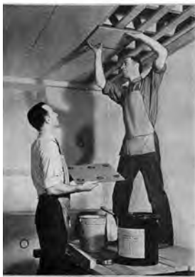
APPLICATION OF INSULATING THERMOBOARD TO CEILING BY MEANS OF AN AIR-BLAST
