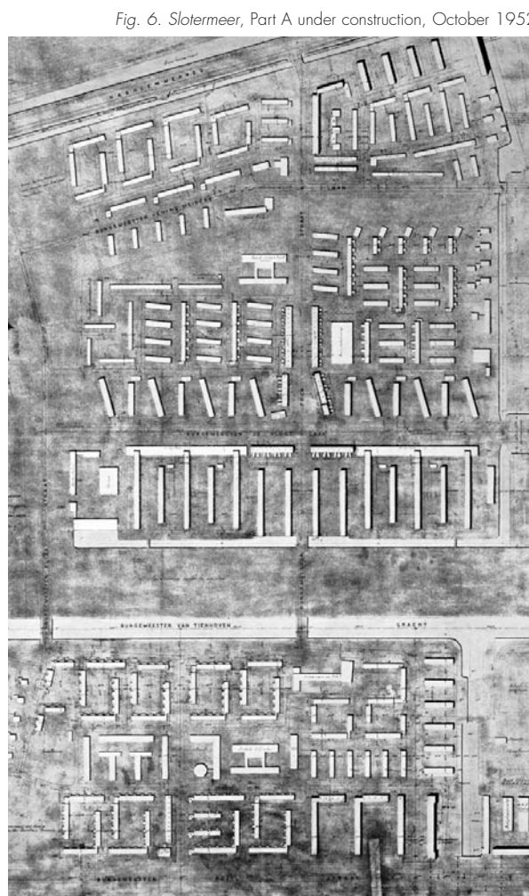
Fig. 6. Slotermeer, Part A under construction, October 1952
