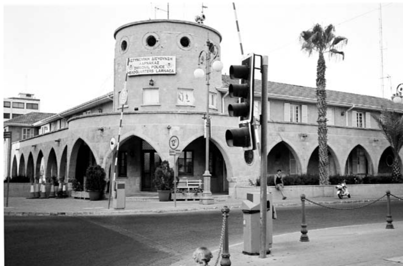
Fig. 1. Front facade of the colonial police station in limestone. The rationalistic style is combined with a traditional architectural idiom
