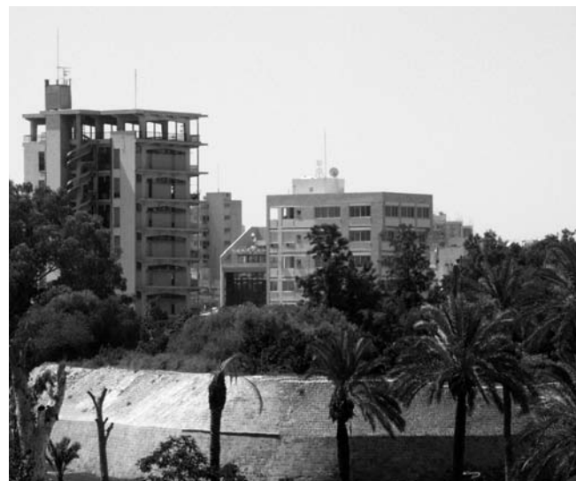
Fig. 7. Neoptolemos Michailides, Demetriou apartment building (poly-katoikia), view overlooking the Venetian walls of Lefkosia, c. 1965
