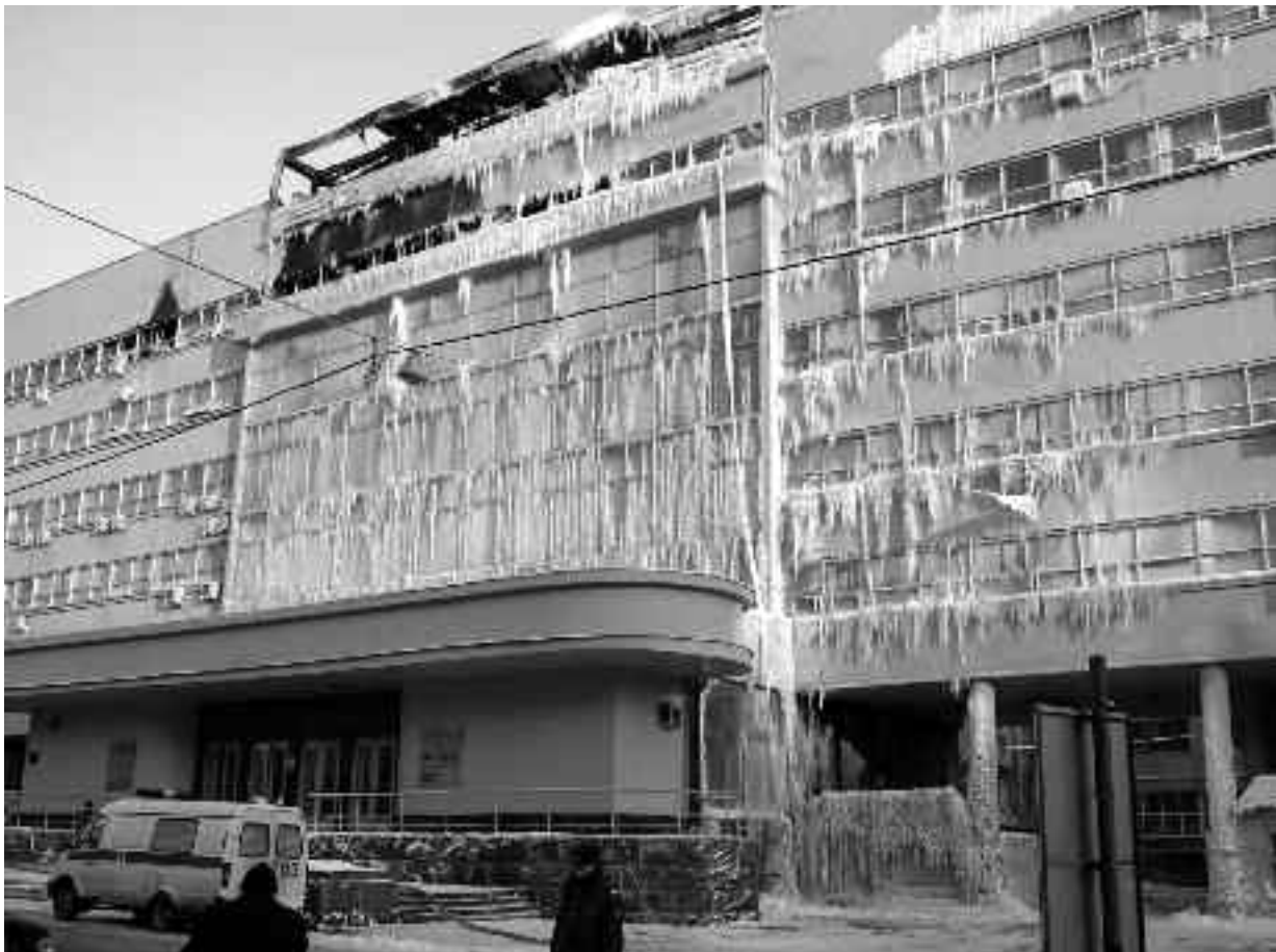
Fig. 7. The Pravda Publishing House, front of the editorial building on the Pravda Street just after the putting out of fire. On the top floor, the middle share or the roof frame is collapsed. Photographed on February 2006
