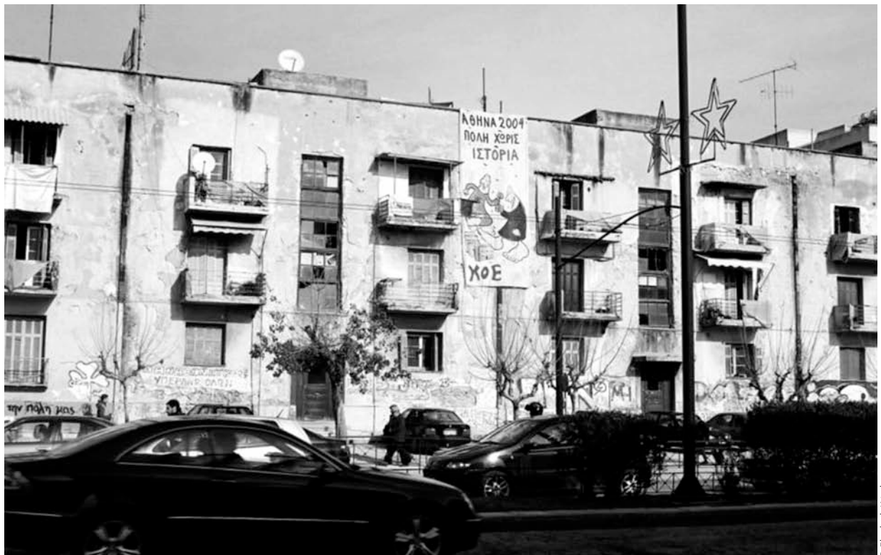
Fig. 4. Façade looking on Alexandras Avenue with a tarp representing the Olympic mascots demolishing the complex, January 2004
